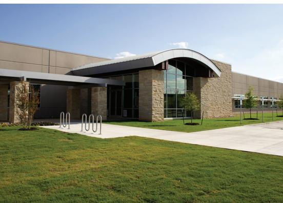
▲ HDA Architects recently completed a 420,000-square-foot distribution center for Capitol Wright Distributing, which features insulated concrete tilt-up walls, high-performance glass and aluminum solar awnings. (Image courtesy of HDA Architects)
